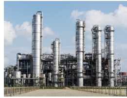
Oil and gas pipeline surveillance
